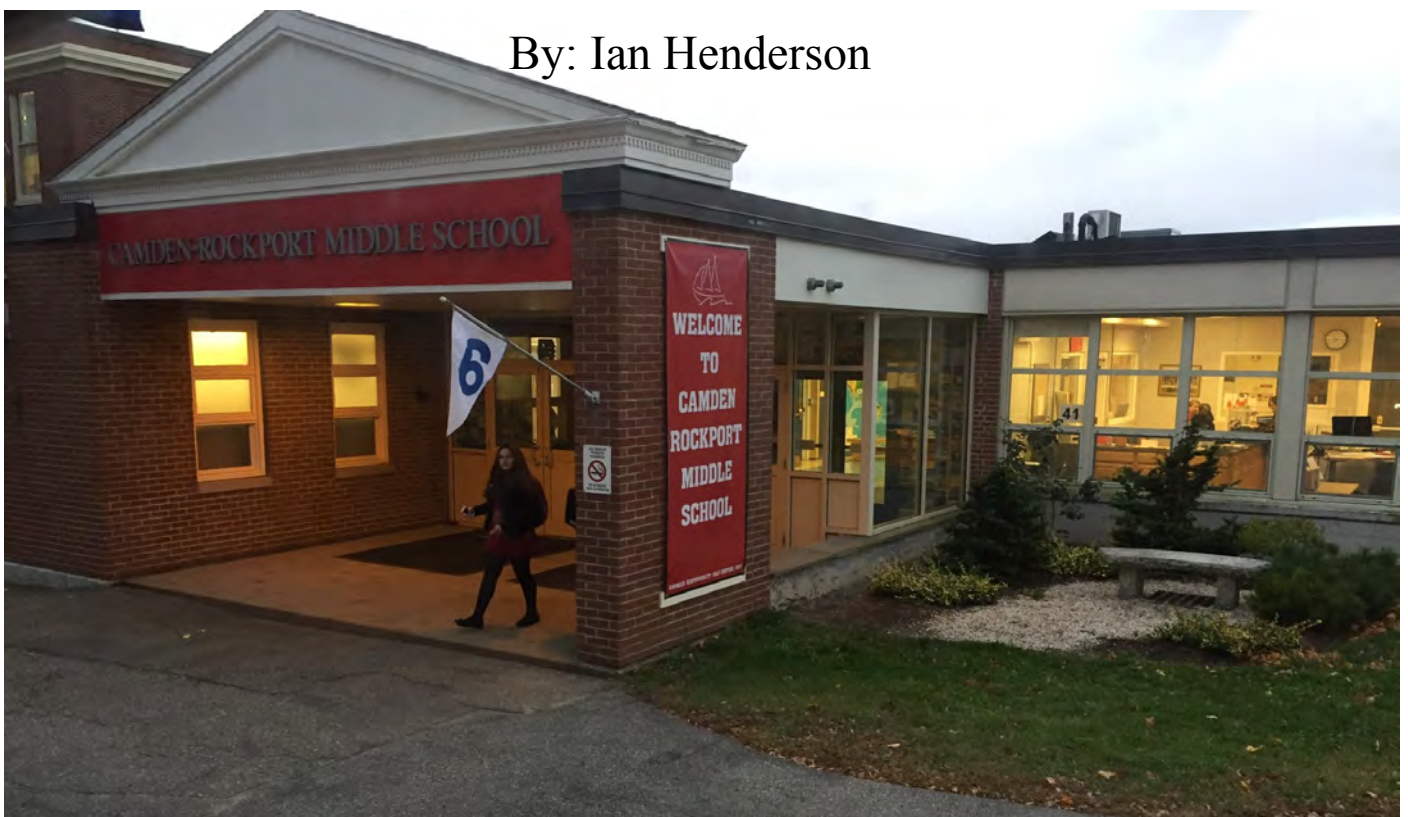
The red brick entrance leading into the slowly decaying Camden-Rockport middle school.
